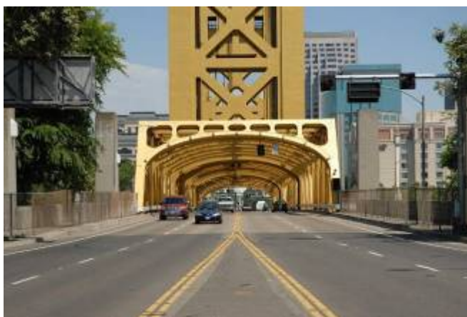
Figure 14. West Sacramento Approach to Tower Bridge
